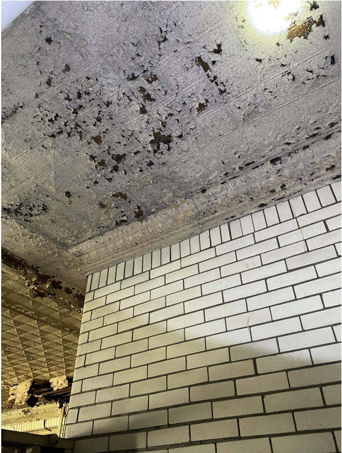
13. Lower story interior showing tiled walls and metal ceiling.
