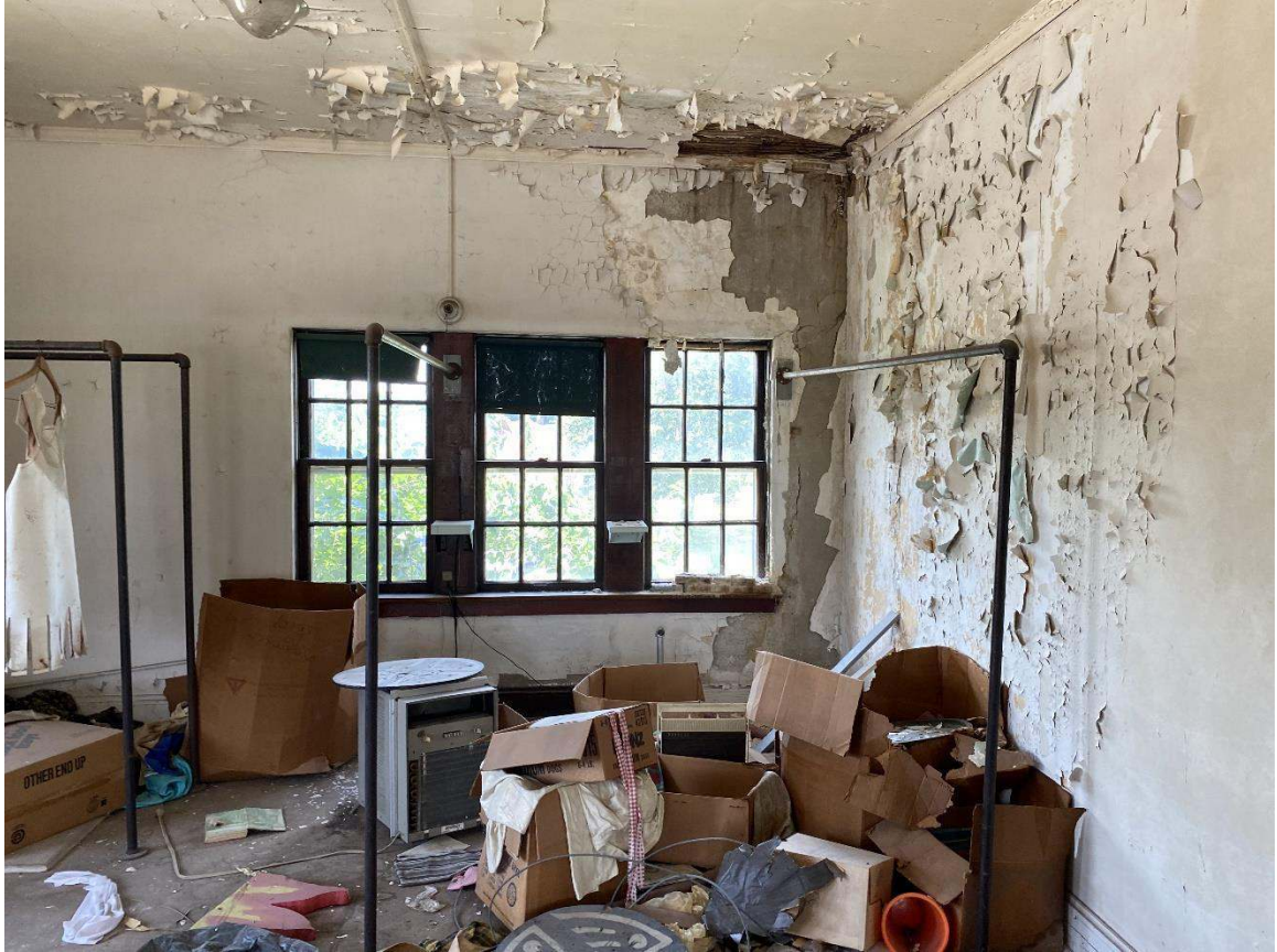
5. Upper story interior showing sleeping quarters.
