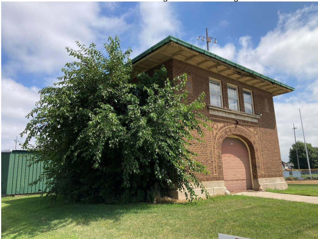
2. View of the west and south building elevations looking from the southwest.
