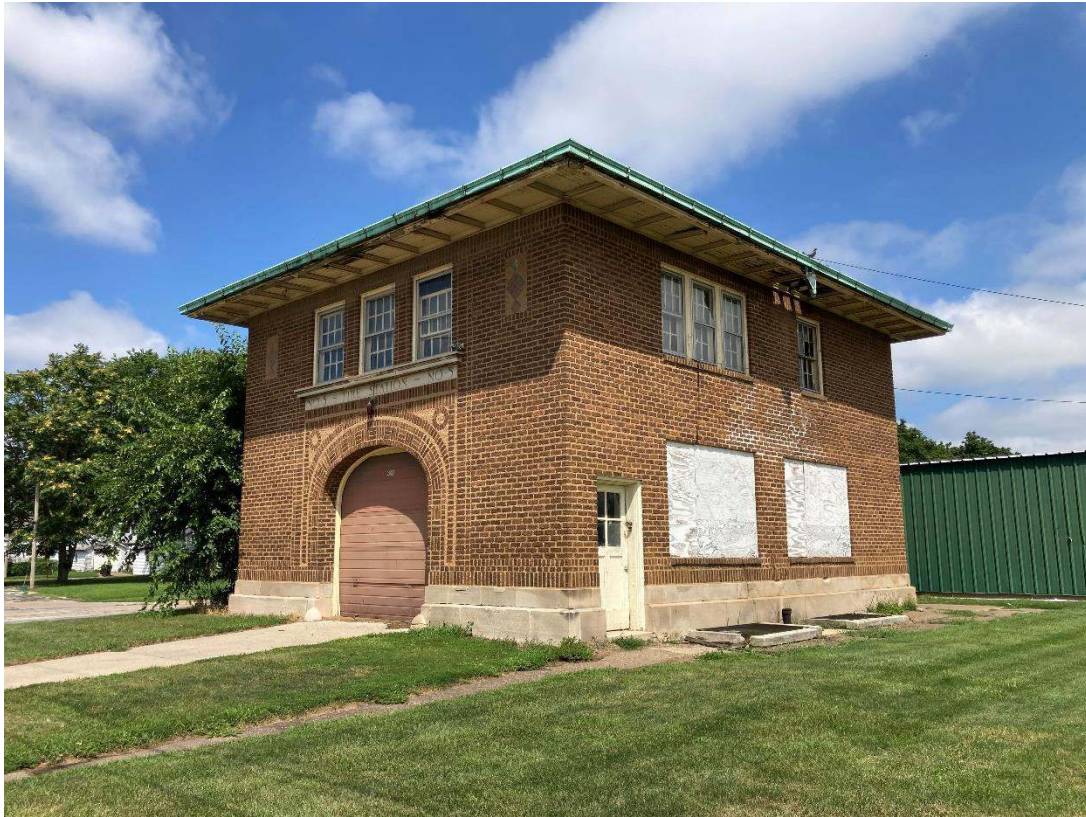
1. View of the south and east building elevations looking from the southeast.
