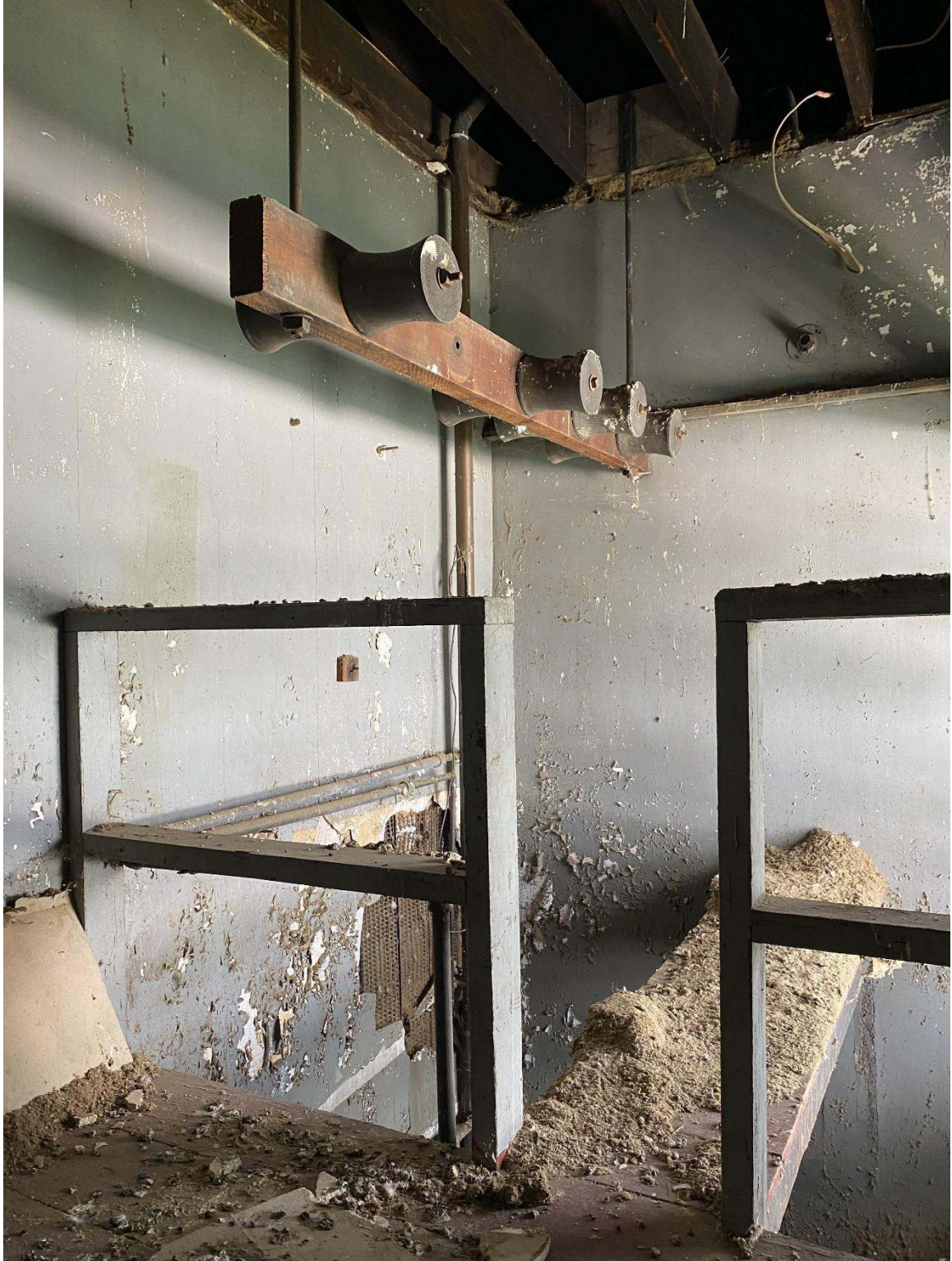
6. Upper story interior showing top of hose drying shaft.
