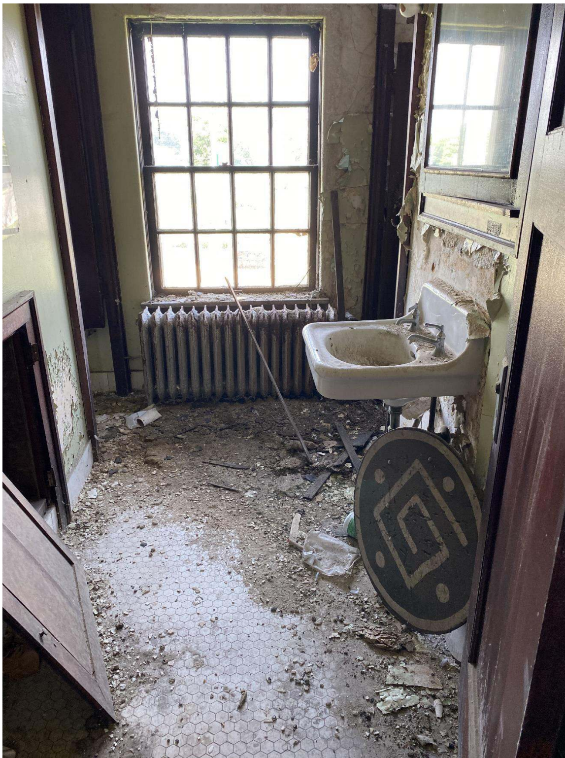
10. Upper story interior showing bathroom.
