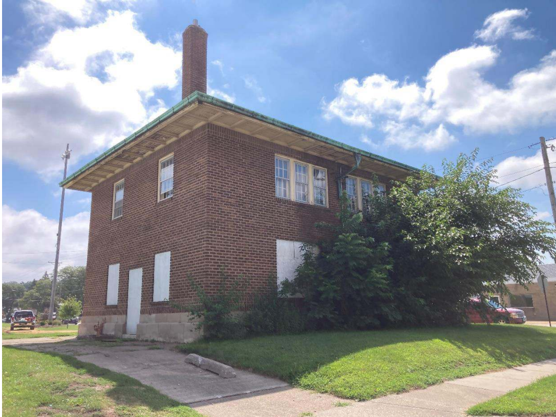
3. View of the north and west building elevations looking from the northwest.
