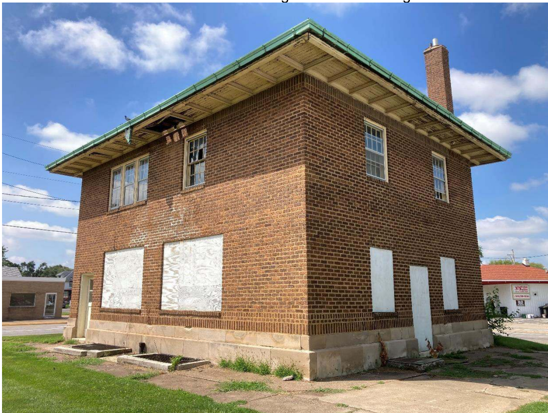
4. View of the east and north building elevations looking from the northeast.
