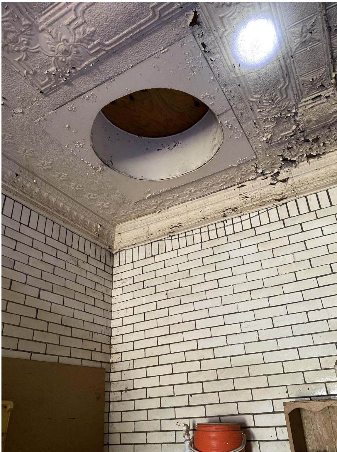
14. Lower story interior showing where a fire pole used to be.
