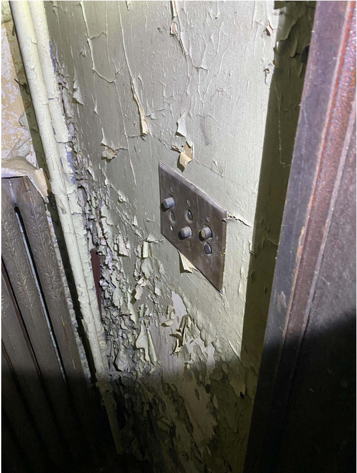
12. Interior stairwell wall.
