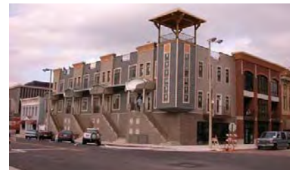
Construction of the Clipper Condos, Rock Island
