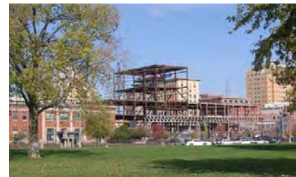
Construction of the Figge Art Museum, Davenport
