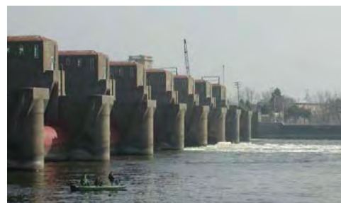
Lock and Dam 15
