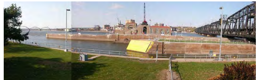
Lock and Dam 15
