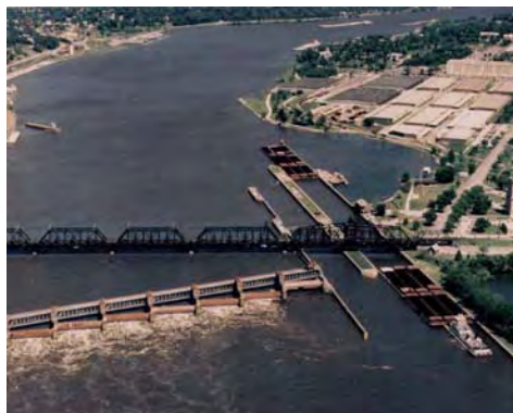
Lock and Dam 15
